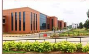
Bangalore, India Receiving Plant
