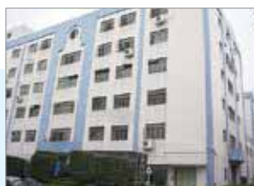
MEAN WELL GUANGZHOU TIANHE R&D CENTER
