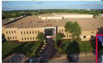
Lincoln, Nebraska Sending Plant
